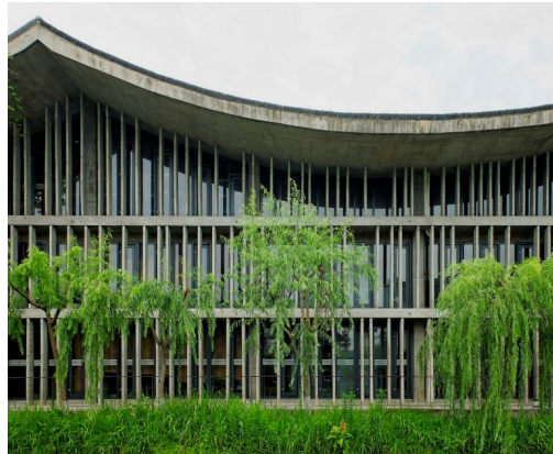
Fig. 12. The campus building of the Xiangshan School of the Chinese Academy of Arts in Hangzhou
