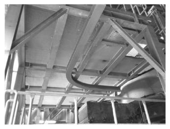
Fig. 1. An example of realization of a curve on plane hoist beam in a industrial plant (photo: author)
