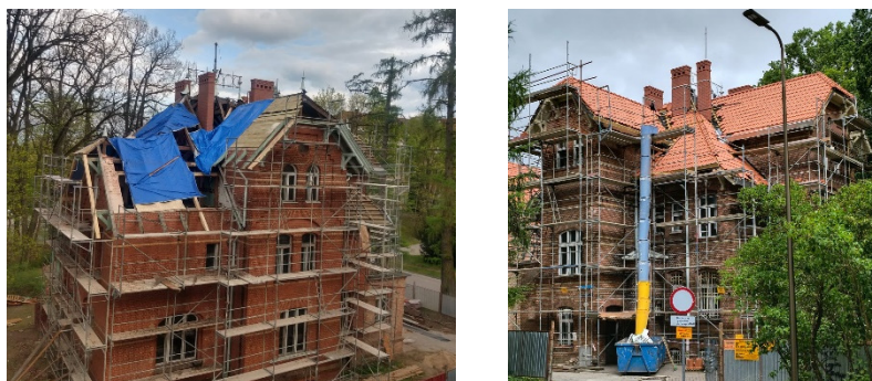
Fig. 2. View of a 19 th -century historical building during revitalization works
