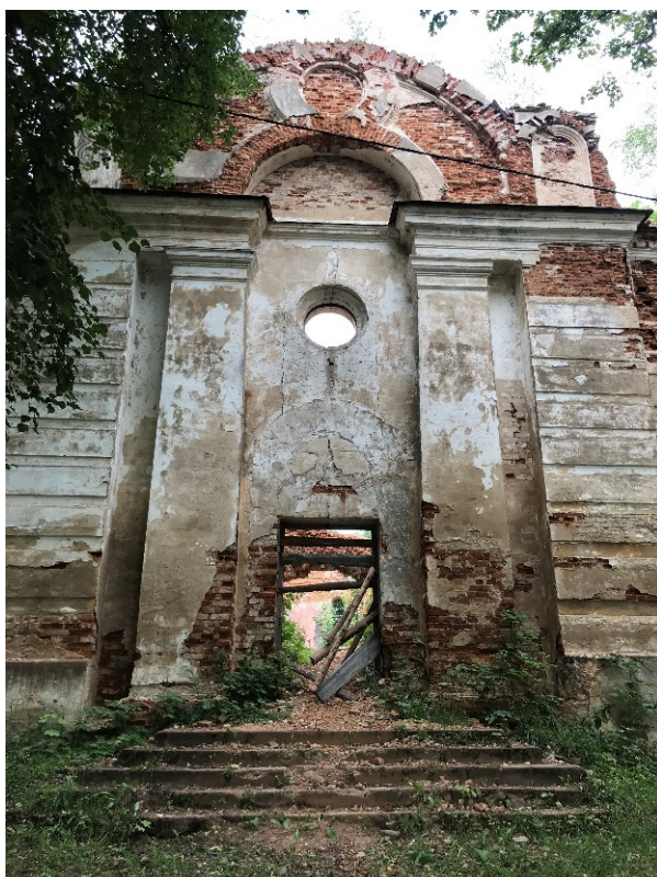
Fig. 1. Church of the Ascension of the Virgin Mary in Dubrovo. The main facade of the church (photo by N. Kalasoškaja)
