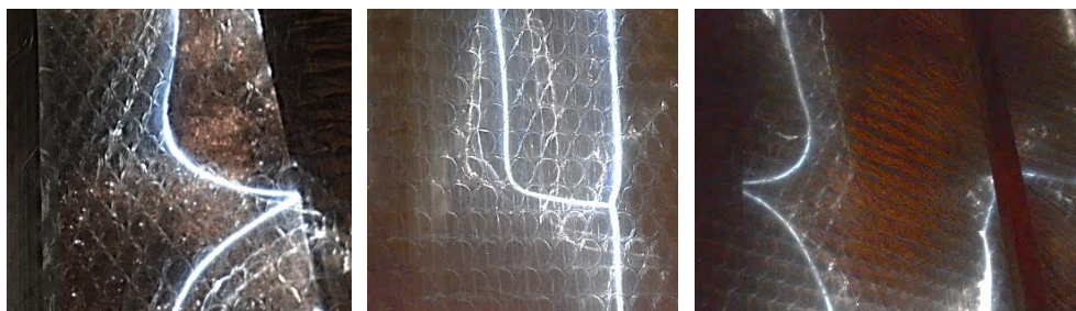
Fig. 3. Cracked glass on the inside
