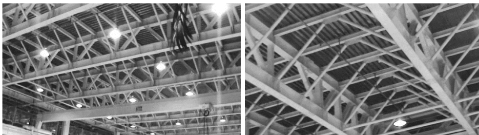
Fig. 5. Roof structure (own photo)
