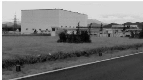
Fig. 4. Above-ground portion of the facility (own photo)
